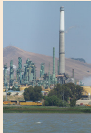
This power plant in Pittsburg uses once-through cooling, which kills millions of marine organisms annually.
